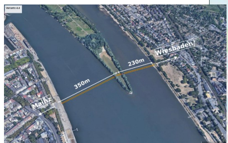
New bridge for cyclists and pedestrians (phase 2)
