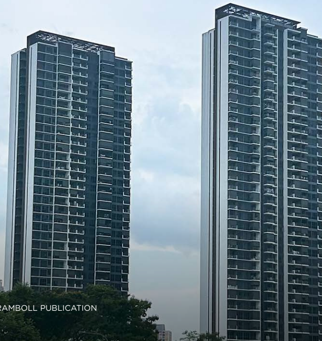
The Clement Canopy (Bouygues Bâtiment International) 65% of the superstructures of two 40-floor tower blocks were constructed using PPVC making it the world's tallest concrete PPVC building.
