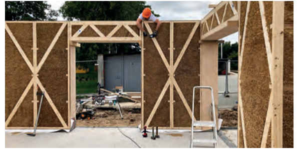
Figure 5 Feldballe School, construction photo
