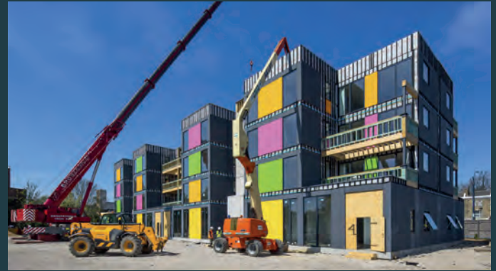
LadyWell Social Housing, Off-site Volumetric Housing
