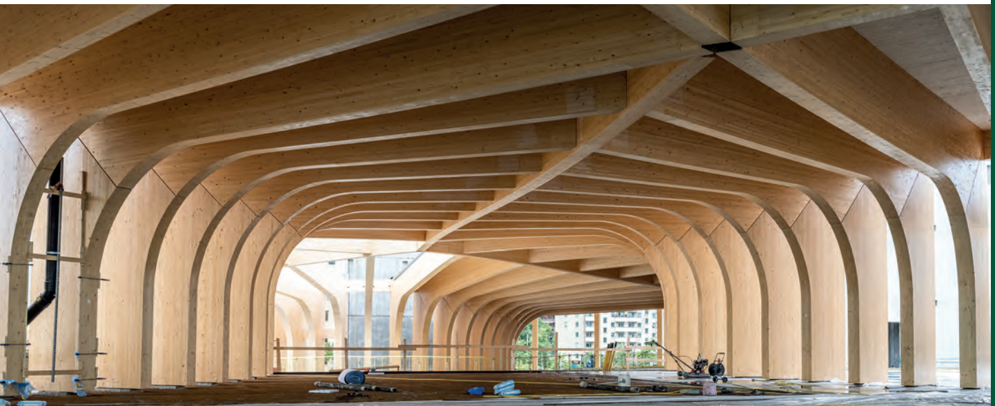
Figure 10 Glulam Beams of World of Volvo Gothenburg, Sweden
