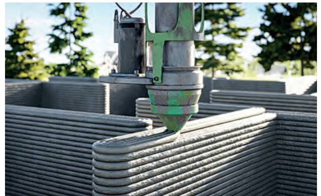
3D concrete printing
