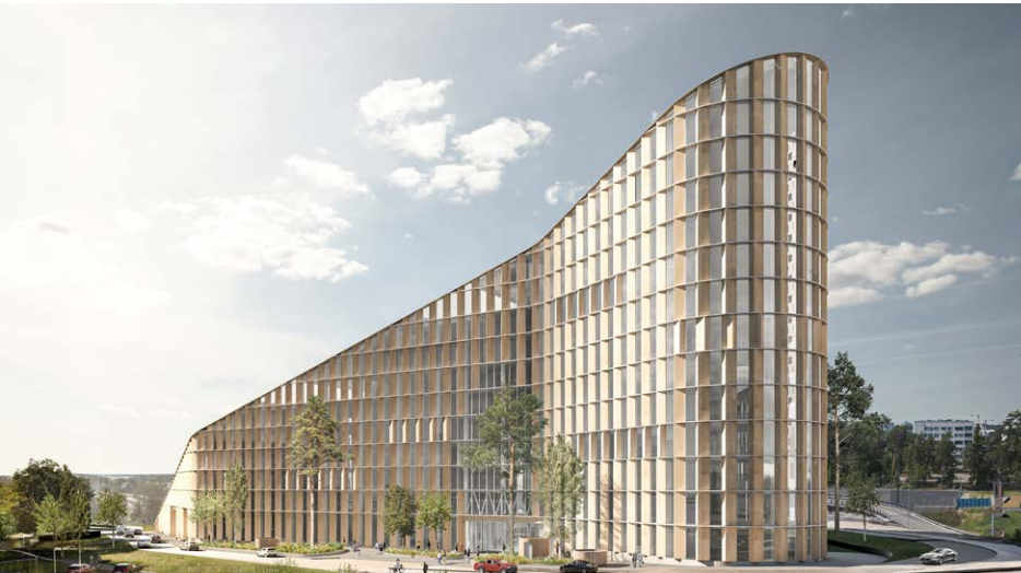
Keilaniemen Portti, Finland (Architects Soini & Horto and Ramboll) Standing at 60m, Keilaniemen Portti will be the tallest timber building in Finland and one of the tallest timber office buildings in the world. The use of timber in the project helped to minimise carbon emissions while enabling a high degree of prefabrication, which reduced the number of deliveries to the site and decreased the number of construction workers required on-site.
