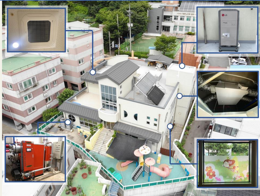
Energy Efficient equipment installed (daycare center)
