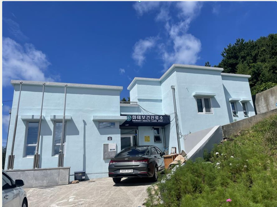
Remodeled Health Care Center
