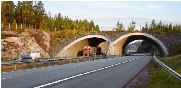
Green bridges helps animals to cross roads safely
