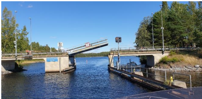
Remote opening of the bridge
